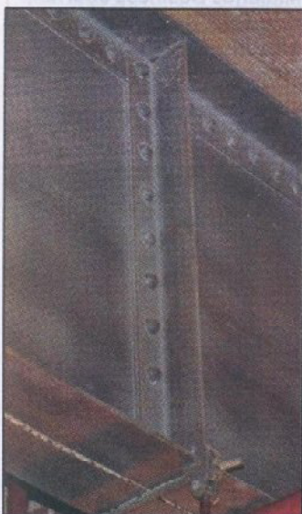
Steel I-beams held by rivets.
